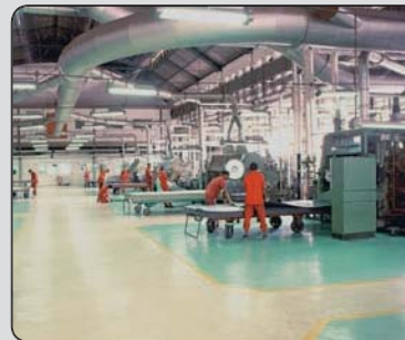
Gasket Sheet Plant
