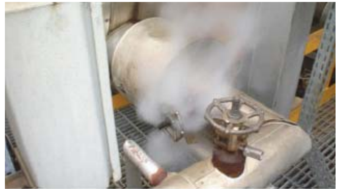
FIGURE 14 – LEAKING VALVE
