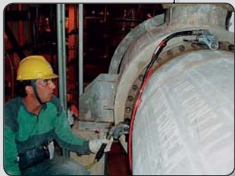
Controlled Torque Gasket Installation
