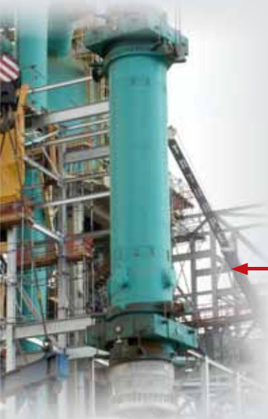
Gimbal Cold-wall Expansion Joint - ID 64 in
